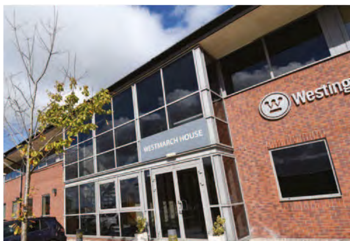
Buckshaw Office Park, Chorley.
