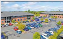
3. Buckshaw Office Park, Chorley
