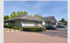
4. Mill House/Mill Court, Milton Keynes
